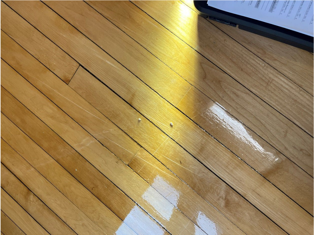
June 9, 2025 - Brown Inspection Photo
